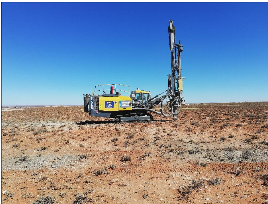
Figure 6: Pre-drilling of holes prior to the ramming of steel piles.
