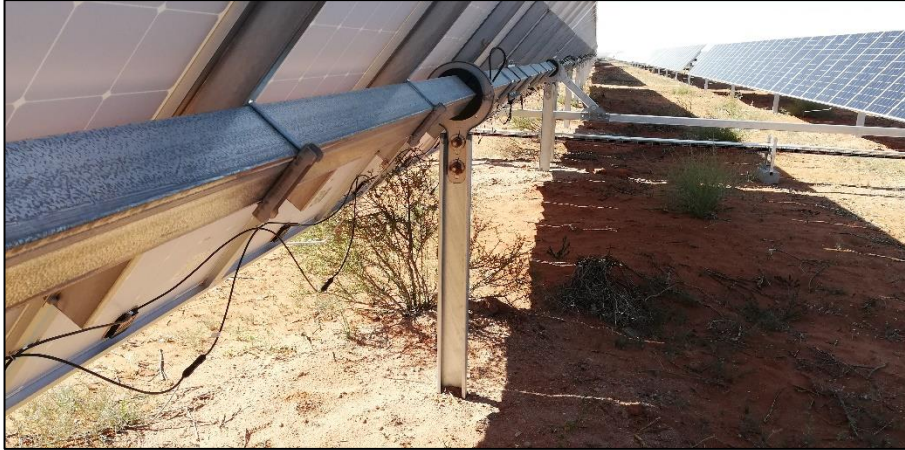
Figure 9: Completed racking and assembly showing vegetation remaining intact beneath the modules.
