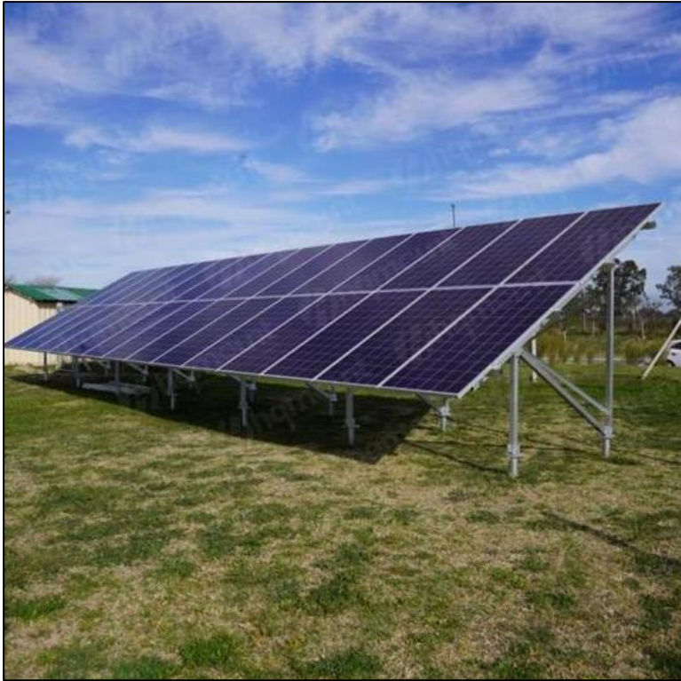
Figure 5: Example of Earth Screw Mounting Technology (HQ, Mount 2023)
