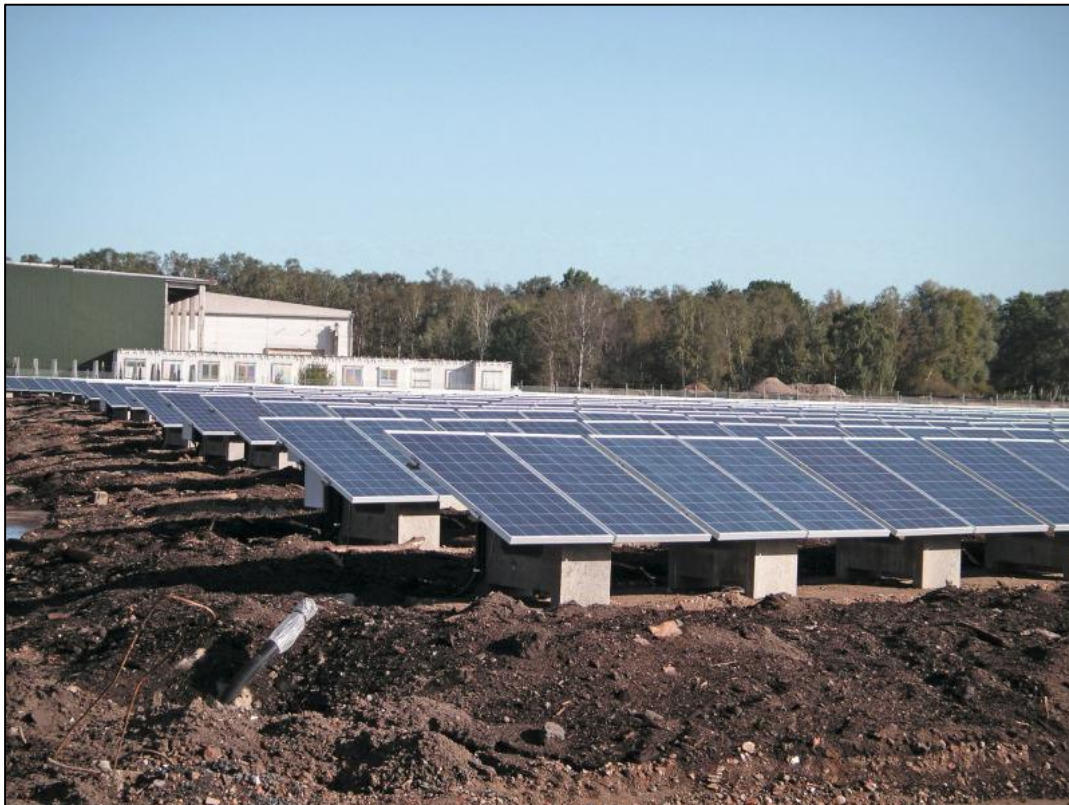
Figure 4: Example of cast concrete mounting systems (BVI International 2023)
