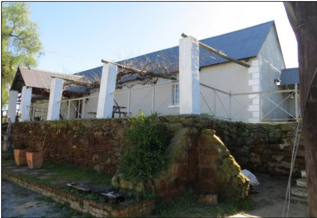
Figure 34: South-eastern corner of the older house on its large stone plinth (waypoint 440).
